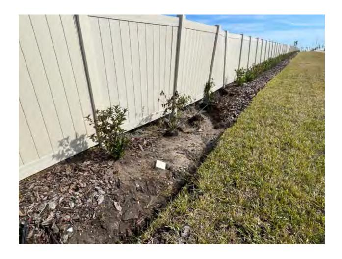
There is a wash-out area on the N.W. side of Berry Grove Blvd that caused the fence damage. This area will need to be regraded. The fence has since been repaired by the contractor responsible for the damage.
